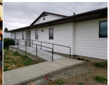
New ADA ramp at north Entrance of home
