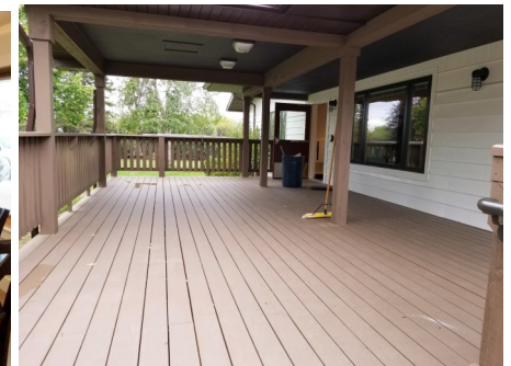
New covered deck is larger and provides better accessibility
