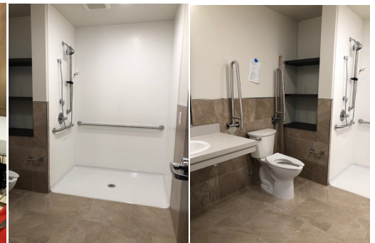
All 4-bathrooms have been completely renovated & are now fully ADA accessible
