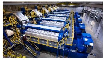
RICE are becoming an increasingly popular choice for utilities. They generally have higher thermal efficiencies than SC-CTs, and efficiency does not vary significantly over the operating range of a single unit. They also offer modularity (ability to add additional units to existing units in small blocks) and quicker start-up and ramp times, are capable of more frequent starts and stops, and help lower operating and
