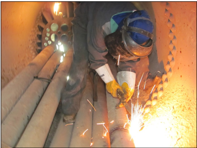
Apprentice Boilermaker Sarah Smith cutting 5" flues into sections for easier removal from boiler.
