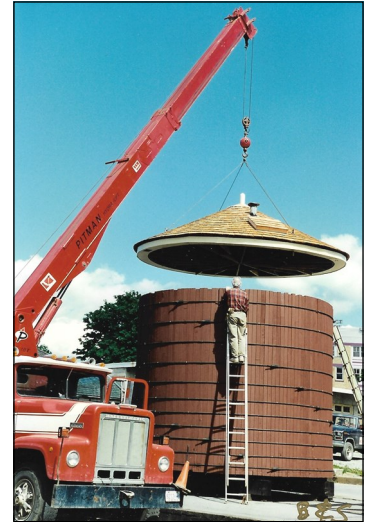
Lifting Roof onto Water Tower at the Train Station— 1996 . "K.G. Campbell" crane does the lift. "Soup's" cranes have made many lifts for us in the 35 years.
