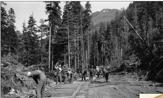
TRACK GANG laying rail into a new logging setting. Heavy work. New immigrants often were given this work. Boyko Sr. could speak 5 languages—an advantage when you were the Foreman.
