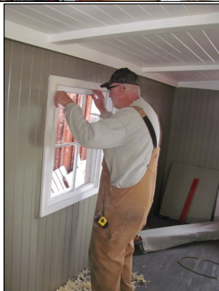
(Above) Sandy Fitzpatrick installs window
