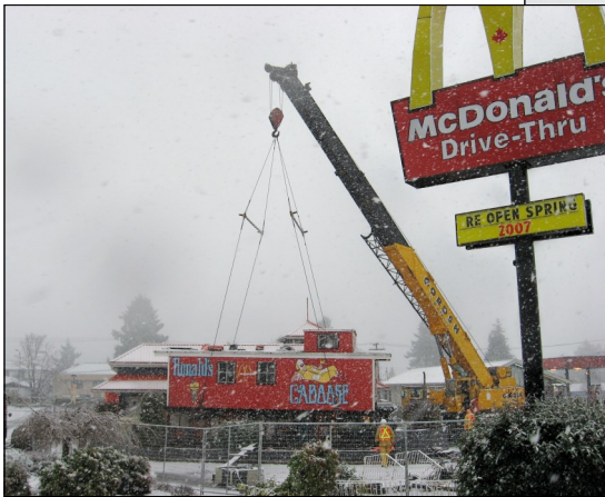
December 2006 Big Lift in Nanaimo Caboose was lifted onto a lowbed.
