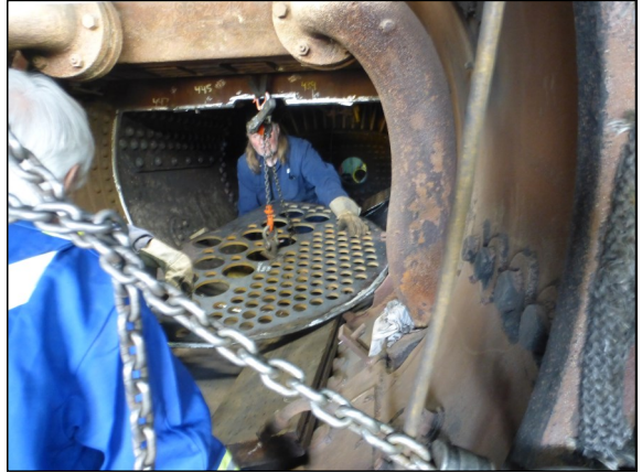
(above) Wrestling a Tube Sheet into the Boiler (left) Rocky checks the fit of the Tube Sheet. (Below) Brent Graham prepares to weld another pass on the Tube Sheet next to the Fire Box.
