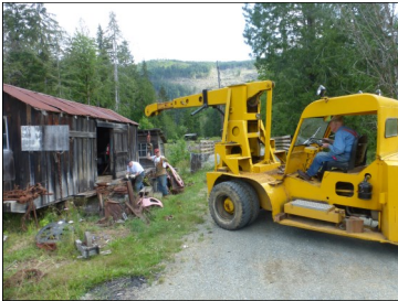
(l.) Replacing planks at Rigging Shed (McLean Mill)
