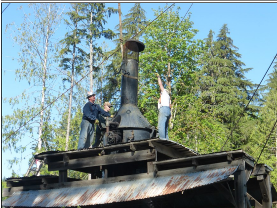
6 Removing the Smoke Stack Photo: D. Hooper
