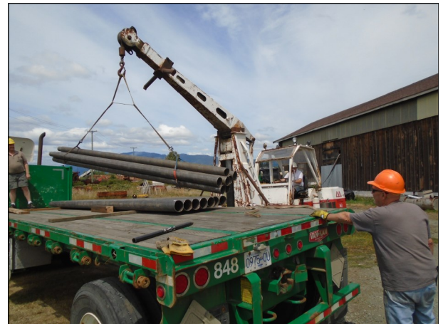
(Below) Pete Geddes supervises the unloading of the 5” superheater flues for the boiler.
