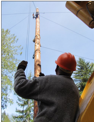
2009 Rigging the Spar Tree Aaron Thom is the Rigger.
