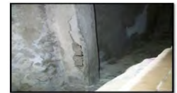
Column Crack
