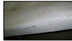
Beam crack
