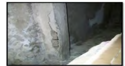
Column Crack
