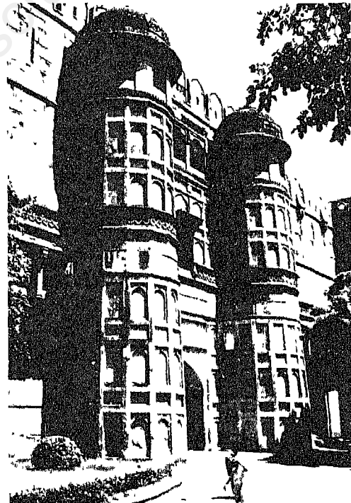
Entrance Gate, Agra Fort
