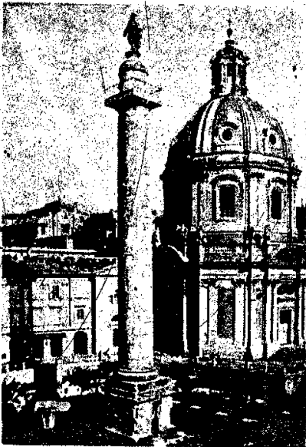
3.24 The Trajan's Column, Rome. The column was built in A.D. 113 to commemorate Trajan's victories.
