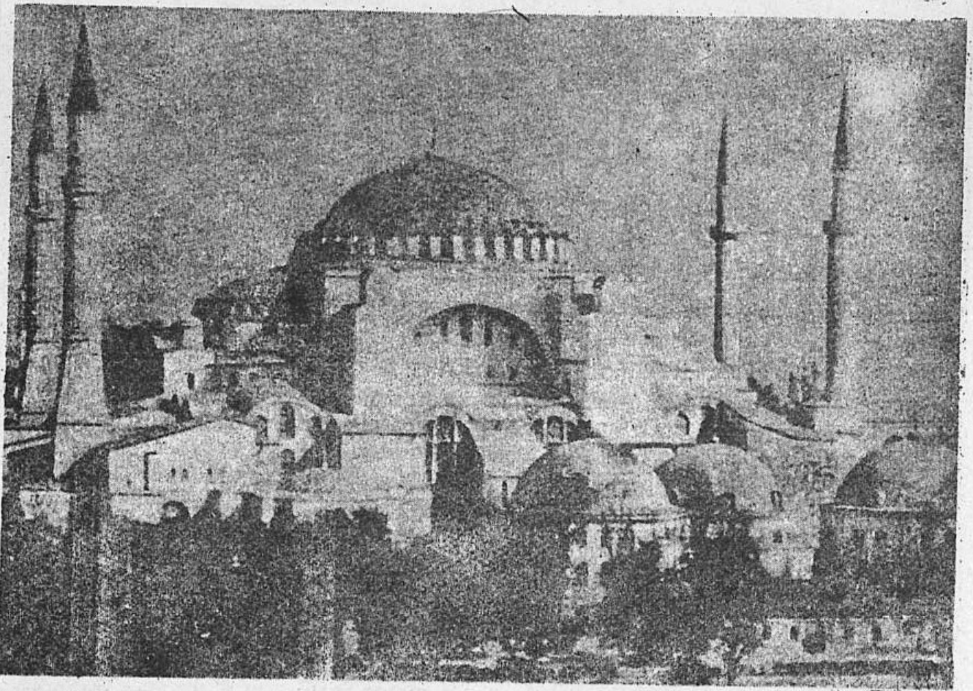
5.1 St. Sophia, Constantinople. The Church was built during the reign of Byzantine emperor Justinian in the 6th century A.D. The minarets were added later by the Turks.
