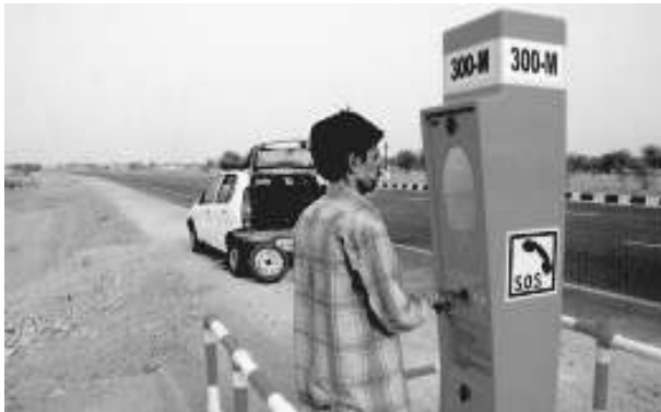
Fig.7.10 : Emergency call box on NH-8
