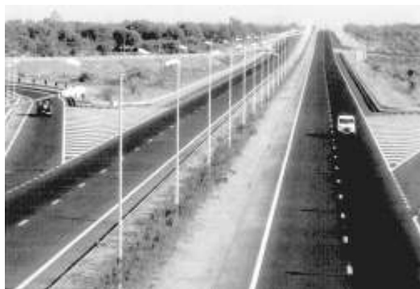
Fig.7.2: Ahmedabad- Vadodara Expressway
