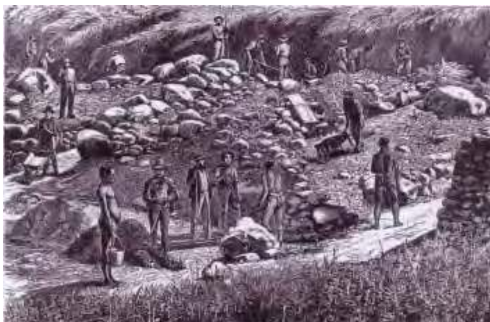
Fig. 13 – Diggers at work in the Transvaal gold fields in South Africa, The Graphic, 1875.
