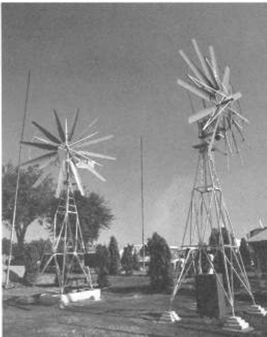
Fig. 8.7 Wind mill : another source of generating power
