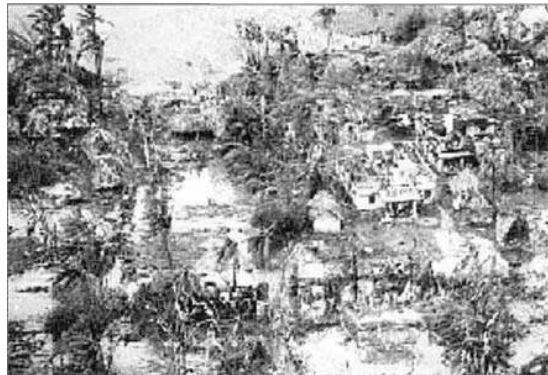
Destruction caused by a cyclone
