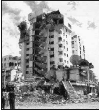
Fig. 3.3a: Destruction caused by an Earthquake in Gujarat
