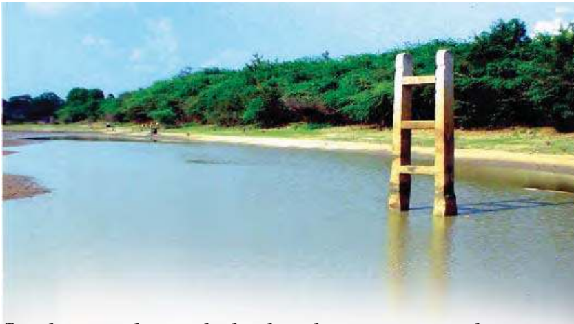
Fig. 5 A ninth century sluice-gate in Tamil Nadu. It regulated the outflow of water from a tank into the channels that irrigated the fields.
