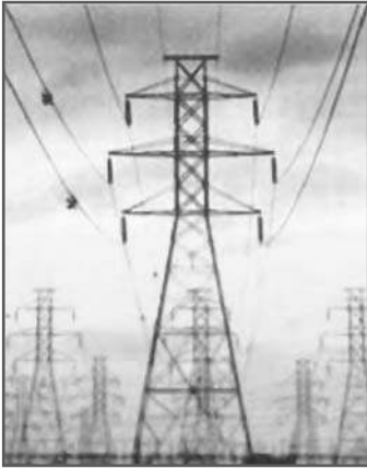
Fig. 3.9: National Power Grid to supply Electricity
