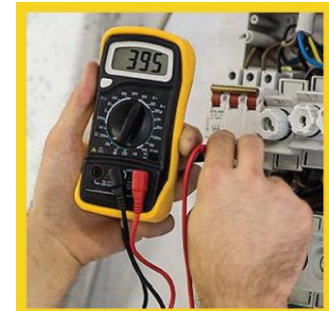
Power Protection & Maintenance Supply
