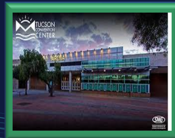
In-Building Neutral Host
