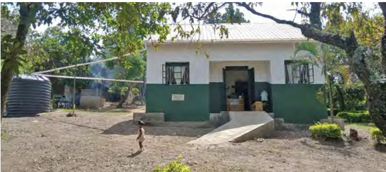
Front view of the renovated Namwasa Clinic, with access ramp
