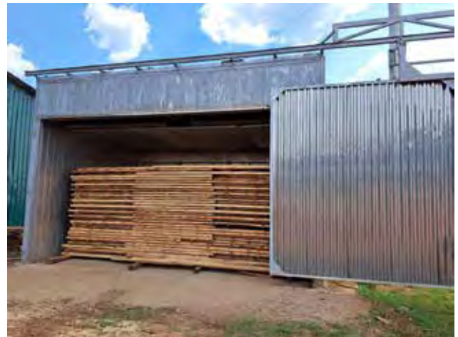
Timber Drying Kiln on site and powered by Hydro Power
