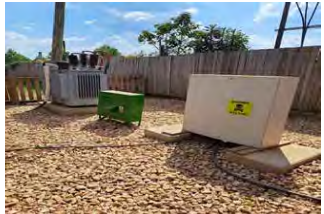
500kV Transformer on site
