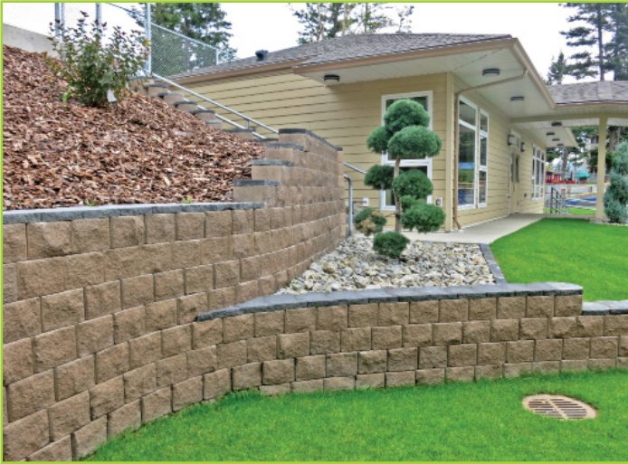
ROCK FACE WALL WITH TERRACES
