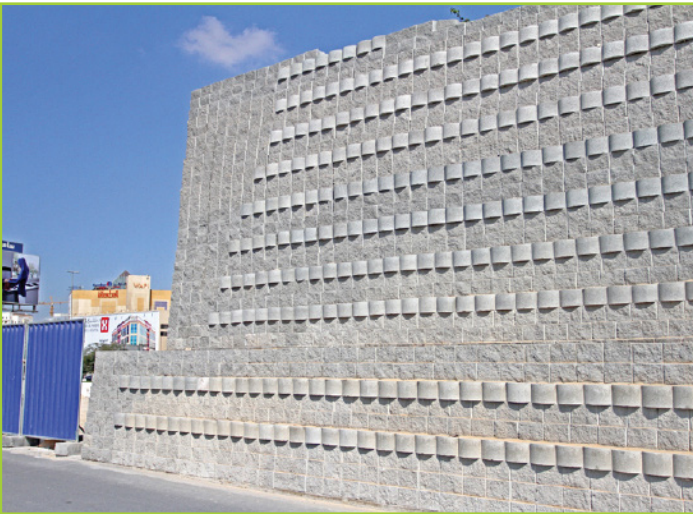
SOUND BARRIER WITH ALTERNATING FINISH
