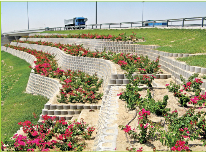
ROCK FACE TERRACES AT AN INTERCHANGE
