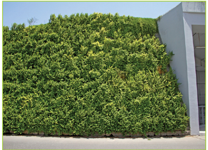
AFTER: PLANTED SOUND BARRIER
