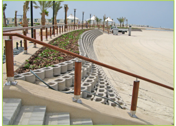
CURVED ROUND FACE RETAINING WALL
