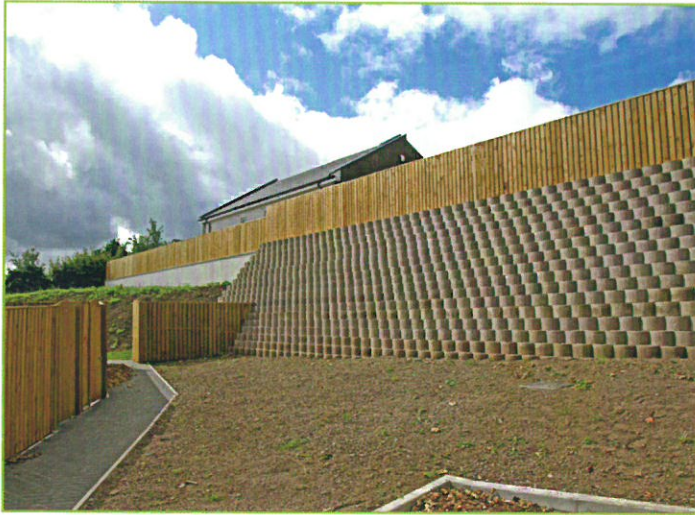
ROUND FACE RETAINING WALL
