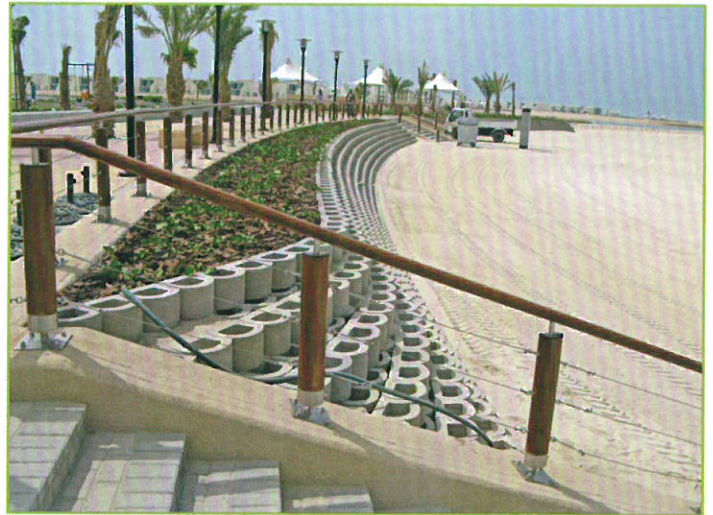
CURVED ROUND FACE RETAINING WALL
