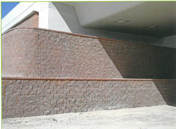
RETAINING WALL AT A HIGHWAY INTERCHANGE
