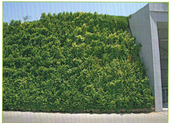
AFTER: PLANTED SOUND BARRIER
