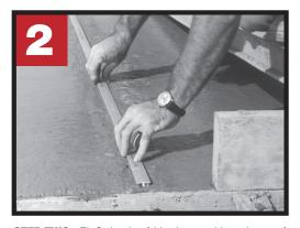
**STEP TWO:** ZipStrip should be inserted into the newly created void so the horizontal portion, top section of ZipStrip is flush with the surface of the concrete.
