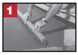
**STEP ONE:** A straight edge or other type of thin bladed material can be used to separate the aggregate in freshly poured on-grade slabs. The aggregate can be separated by using a back and forth motion approximately 2" deep.
