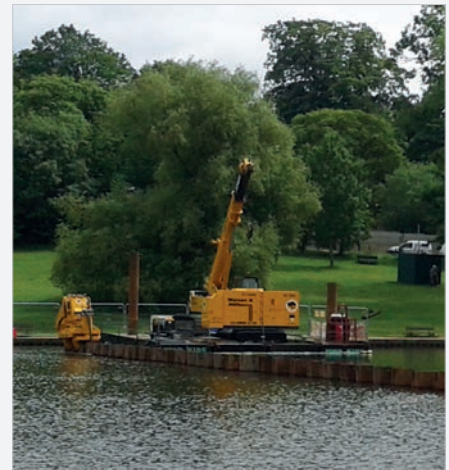
Work over water
