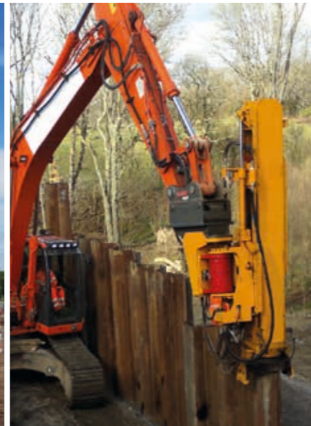
DX-SP DRIVING SHEET PILES
