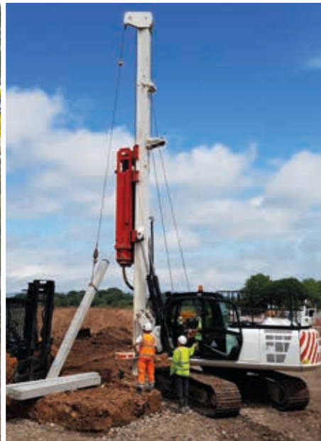
DX HAMMER MOUNTED ON JX25-8 PILING RIG
