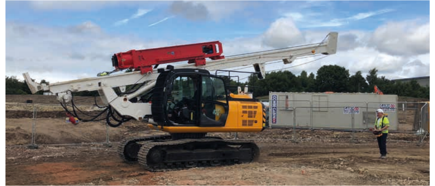
RIG BEING OPERATED BY RADIO CONTROL
