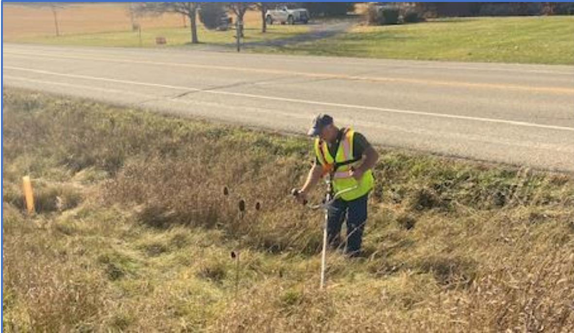
Figure 11 Stripping vegetation using brush trimmer. Elmira ON. November 2022
