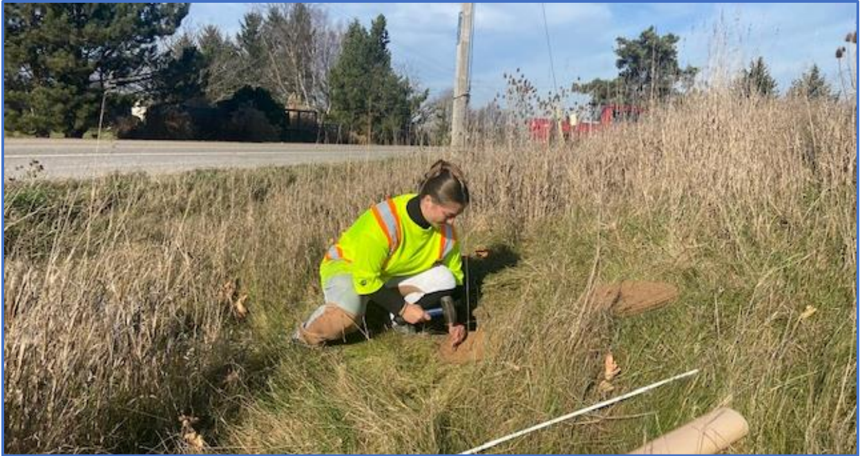
Figure 13 Installing coco fibre mat. Elmira ON. November 2022
