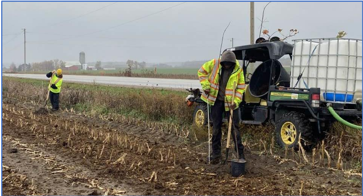
Figure 6 Installing 2 Gallon and 3 Gallon Trees Along Floradale Road, Elmira, ON. October 2022
