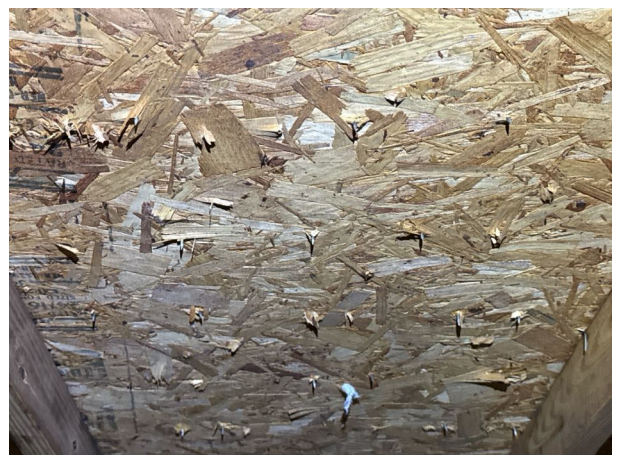
6 Nails Per Shingle From Roof Underside
