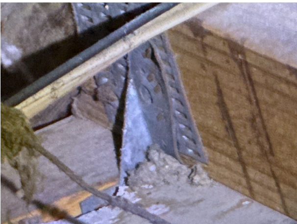
Hurricane Clip Roof To Wall Attachment
