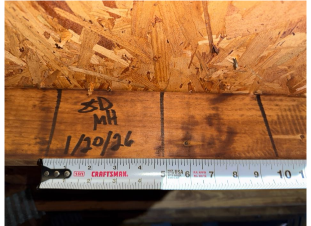
8d Nails Spaced 6" by 6"
