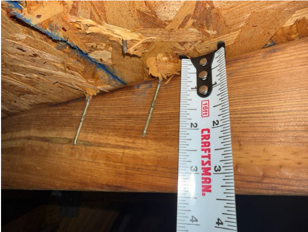
8d Nails Used For Roof Deck Attachment
