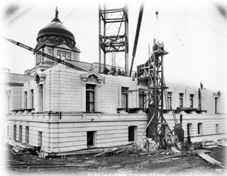
Capitol building construction (1910)
