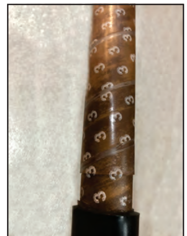
Oil barrier sleeve - PILC cables
