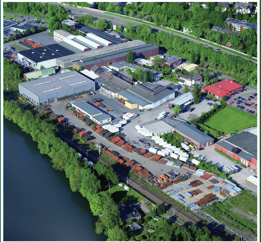
Headquarters of Carl Hamm in Essen, Germany
