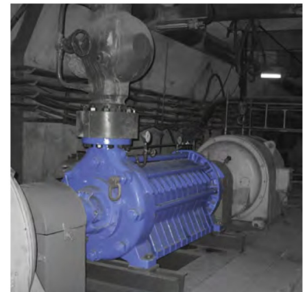
Intermediate flange at stage casing
